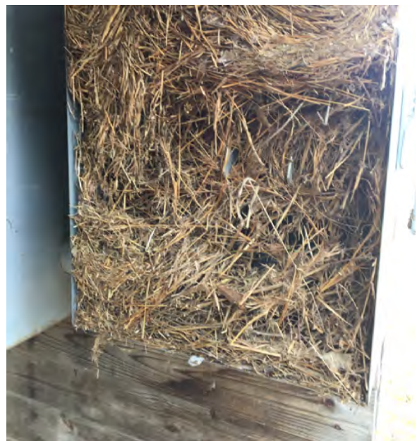
Figure 2: Neglected disconnect
