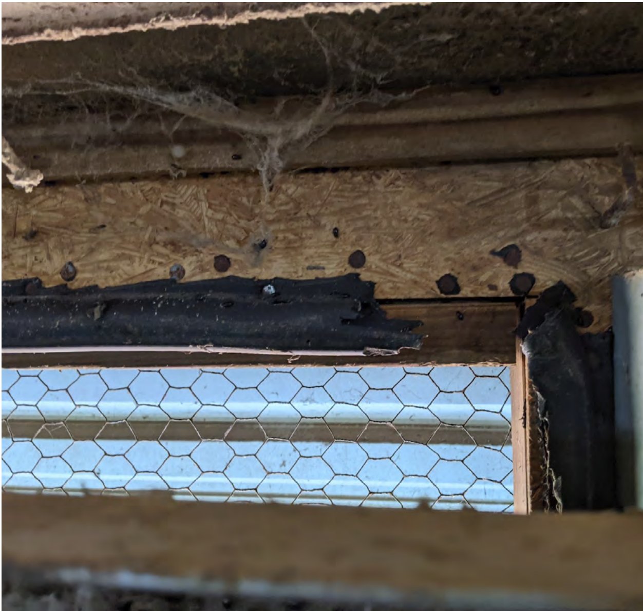
Photo 3: All vent door seals must be inspected and repaired now so they are working for you and not against you in the form of non-uniform air temperatures, cold chicks and excessive heat zone runtimes. Correct vent door air leaks.
