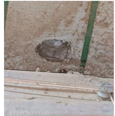
Photo 1: Rat and other holes in the ceiling allow hot air to exit the building and run up fuel bills. Fuel burned to compensate for these air leaks works against your bottom line. We need to rethink our rodent control program here as well.
