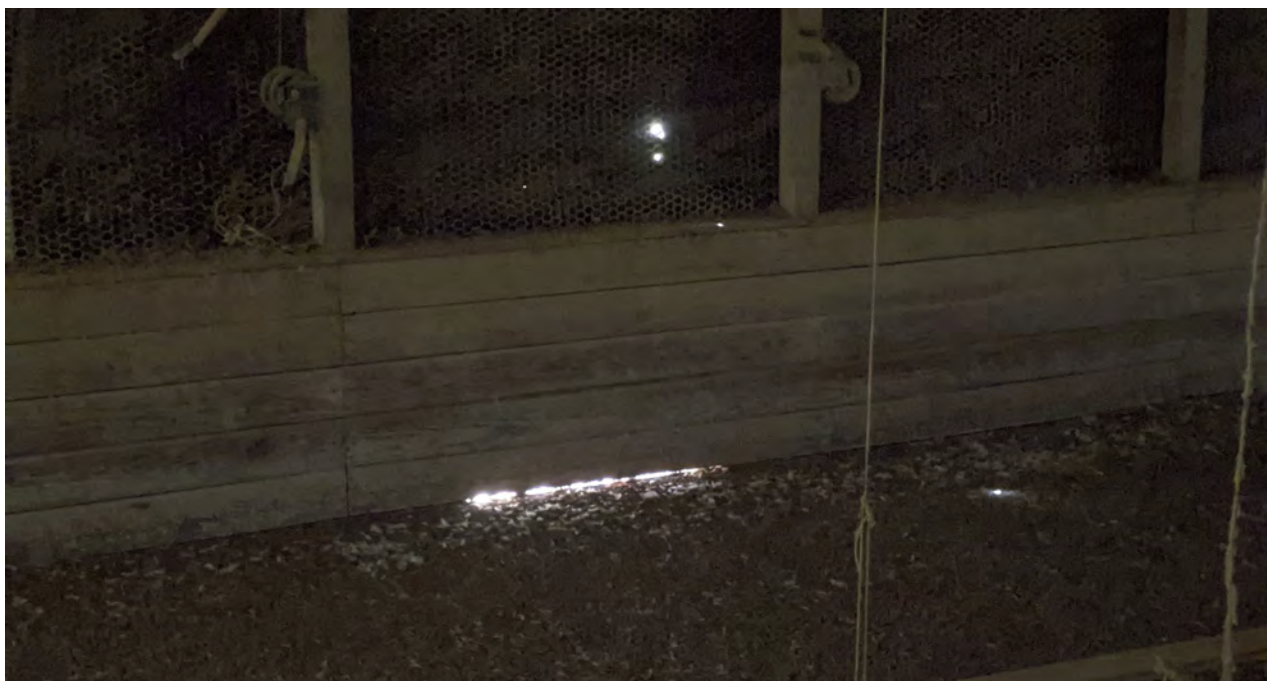
Photo 2: It is hard to run a good offense when your opponent is breaking through the line of scrimmage every play. Block these curtain leaks with some heavy-duty curtain tape and the lower wall with some lumber and caulking or expanding foam. The foam must be protected from bird and beetle damage. At the least, kick some litter back over the hole for a temporary fix.
