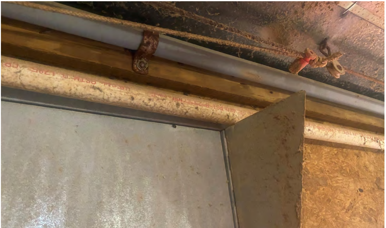
Photo 3: Can you spot this potential friction failure? This is not an example of a moving steel rod, cable or rope. Gravity and friction play a leading role in how this scenario will play out. Regardless, it is just a matter of time before this metal vent shield rubs a hole into this PVC water line and causes major problems inside the poultry house. Again, the goal is to prevent the potential for any and all friction failures from causing problems.
