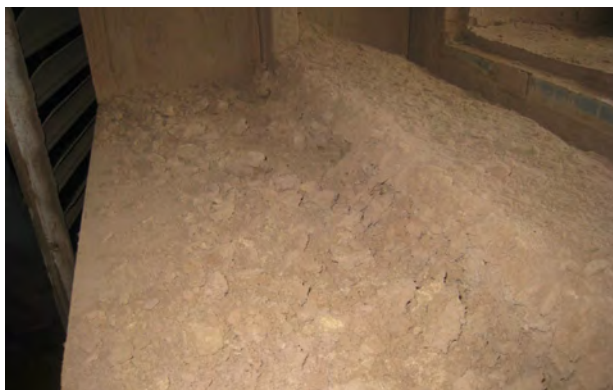
Figures 5 and 6: These photos were taken from a pullet house that was only 5 years old. We are pretty sure the light traps, shutters and fans had never been cleaned. There was about 0.25" of dust on shutters, and about 2.5"-3" of dust settled in the bottom of the light traps and framing. Light traps were totally coated in dust, and about 1-1.5" of dust was in the fan housing. This is a personal foul.
