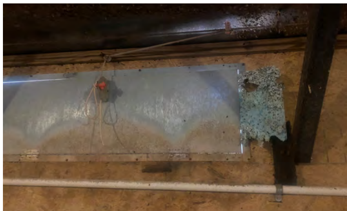
Figure 3: The insulation in this inlet door has almost totally disintegrated due to darkling beetles. This vent is another major source of air leakage and is made worse by the insulation settling out of the door and getting wedged between the door and frame. The metal door appears to be in good shape, so we would recommend replacing the insulation on this door. This was not staged.
