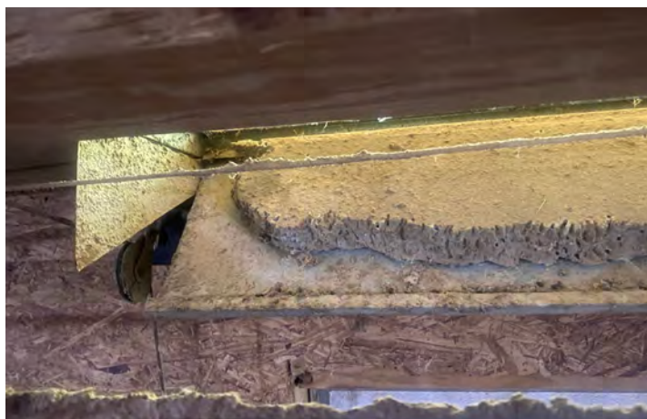
Figure 2: This inlet door is a considerable source of air leakage when shut. The insulation has been damaged by rodents. The door does open and shut, but when it is shut, it does not seal and is leaking on three sides. It is overdue for repair or replacement. This can often be found on inlets located closest to the feed cross-fill entrance to the house, where rodents have direct access to the house wall and attic space.
