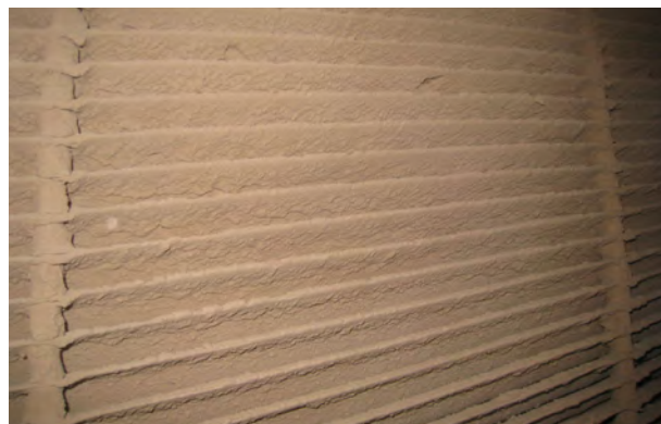
Figures 5 and 6: These photos were taken from a pullet house that was only 5 years old. We are pretty sure the light traps, shutters and fans had never been cleaned. There was about 0.25" of dust on shutters, and about 2.5"-3" of dust settled in the bottom of the light traps and framing. Light traps were totally coated in dust, and about 1-1.5" of dust was in the fan housing. This is a personal foul.
