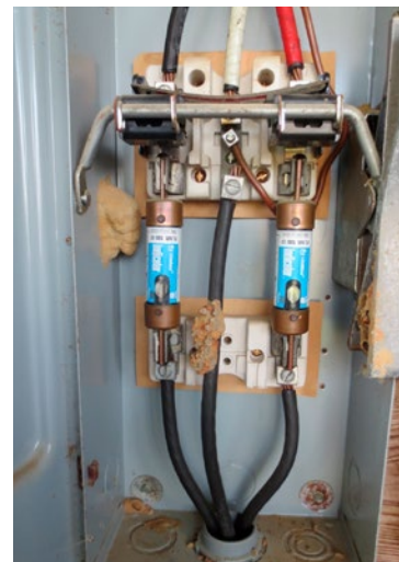
Photo 7: This generator battery is in serious need of cleaning and testing. Can you identify the problem? Photo 8: Each house disconnect will have a breaker or fuse to protect the wires and equipment on the load side. Inspect and clean all these fuses. Can you identify the problem?
