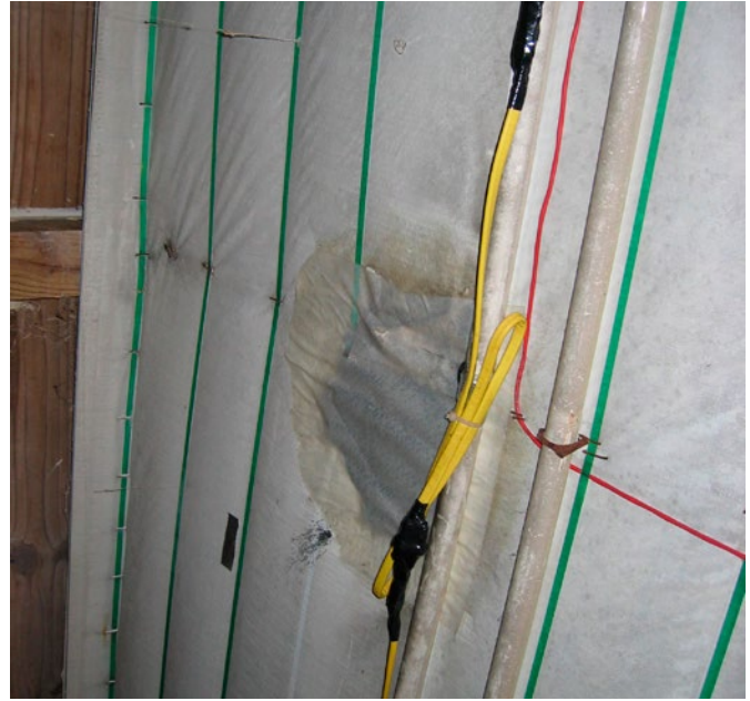
Photo 5: This grower allowed an inexperienced helper to install a new fan circuit and, as a result, nearly burned the building down. Thankfully, we noticed the flame and had access to a fire extinguisher. Photo 6: Not the best repair work we have seen, but the fan works now.
