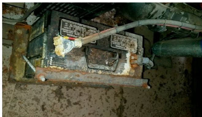
Photo 7: This generator battery is in serious need of cleaning and testing. Can you identify the problem? Photo 8: Each house disconnect will have a breaker or fuse to protect the wires and equipment on the load side. Inspect and clean all these fuses. Can you identify the problem?
