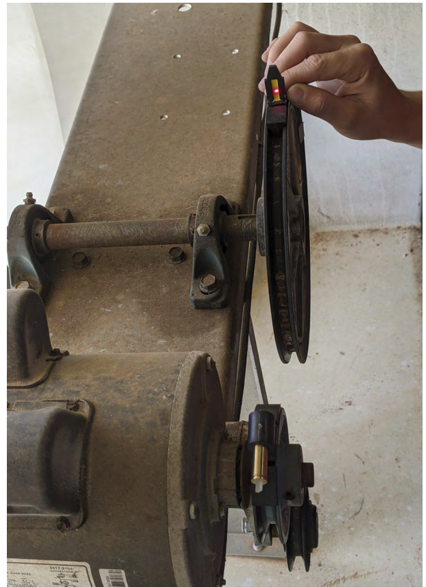
Figure 6: Left photo, the laser method is used on a fan where the pulleys are out of alignment approximately 5/8 inch. Right photo, the laser is hitting inside the yellow acceptable strip, showing the pulleys are in correct alignment.
