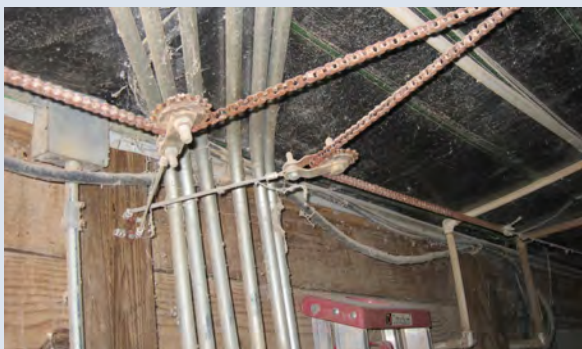
Figure 9: Inlet door chain and sprockets
