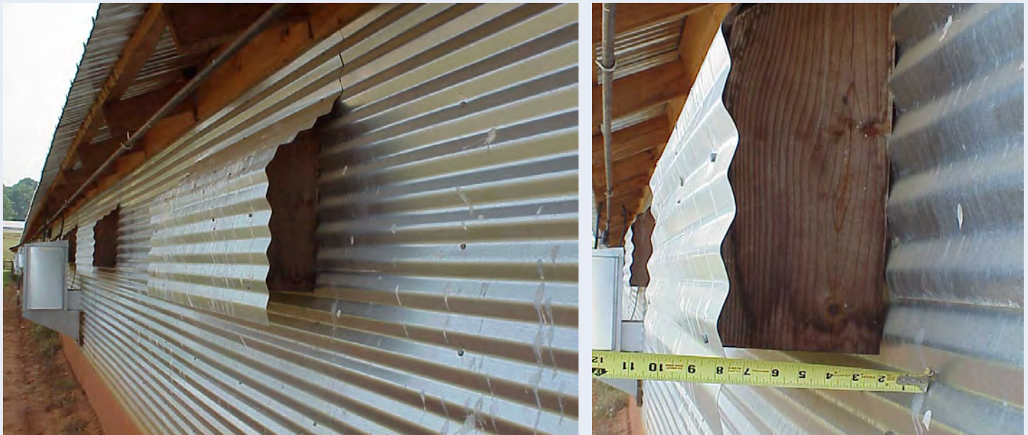
Figure 1: An older example of corrugated metal and framing lumber light shield over perimeter sidewall air inlets in a broiler house. Here we are measuring the size of the opening to see if this shield air opening is properly sized for the inlet it is covering.
