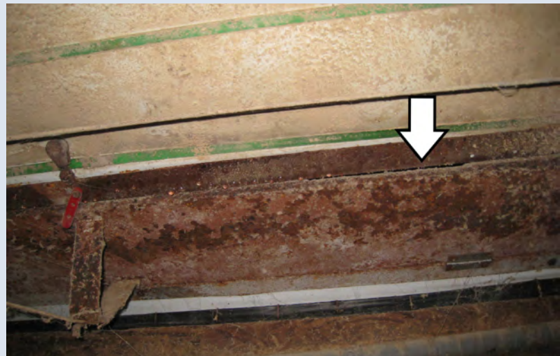
Figure 6: Rusted metal ceiling air inlet door needs to be repaired or replaced.
