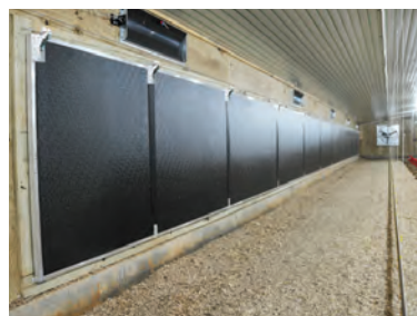
Inside tunnel doors are available in 2', 3', 4', 5', and 6' panel heights.
