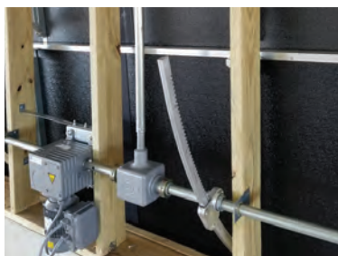
Outside tunnel door drive units can control single, double or triple doors.
