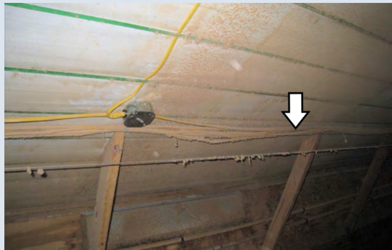
Figure 5: Several romex wires create an obstruction to incoming air from this sidewall air inlet.
