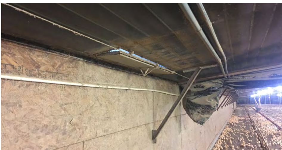
Figure 4: Two electrical conduits running parallel to ceiling air inlets will trip the cooler incoming air stream before it gets a chance to mix with warmer air as it enters the house.
