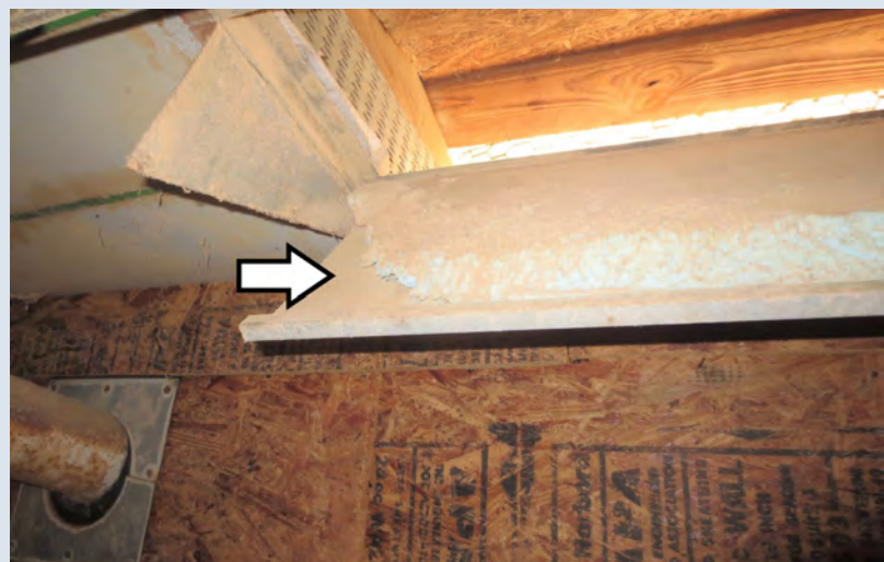
Figure 7: Metal ceiling air inlet door with insulation damaged by rodents, needs repair.
