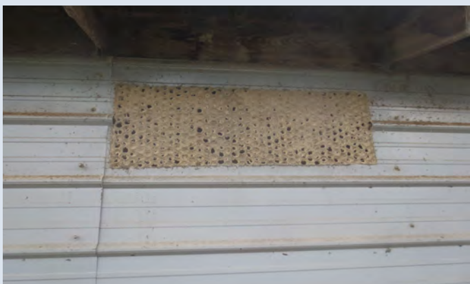
Figure 2: Clogged bird wire over sidewall air inlet.
