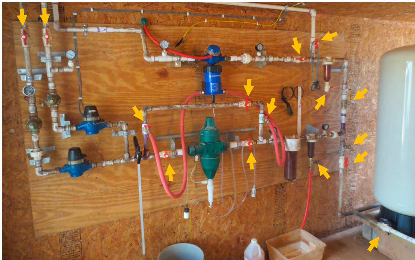
Figure 1: The arrows highlight 15 valves used in this water manifold feeding a 40 x 500 commercial broiler house.
