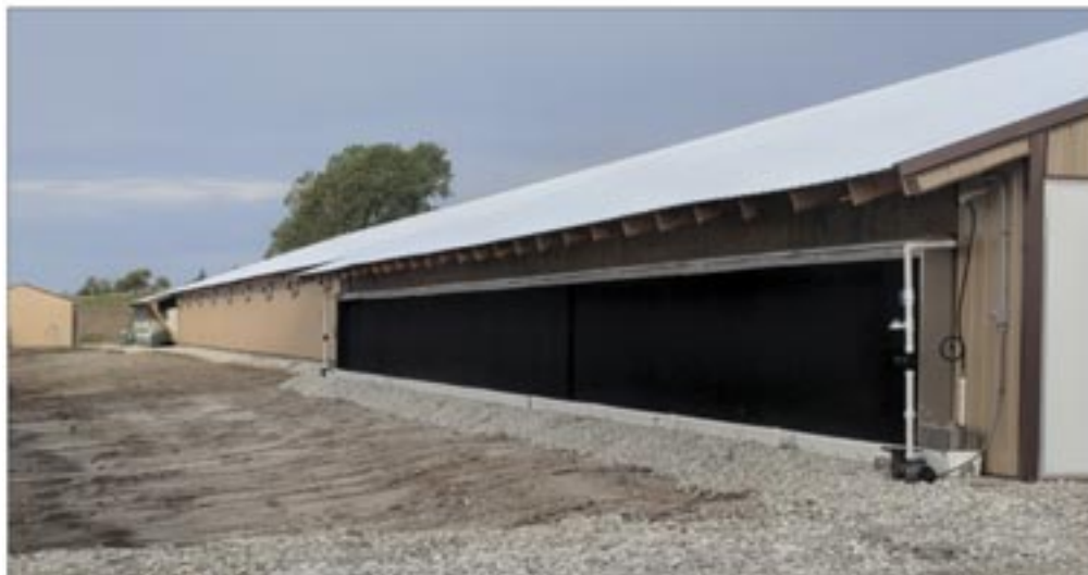
Figure 1. A typical broiler house with an evaporative cooling system and tunnel exhaust fans. The exhaust fans are visible at the far left, while the evaporative pads are in the foreground. This particular system has two pumps on either end of the pads supplying water toward the center.
